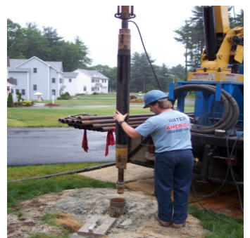
Hydrofracturing
