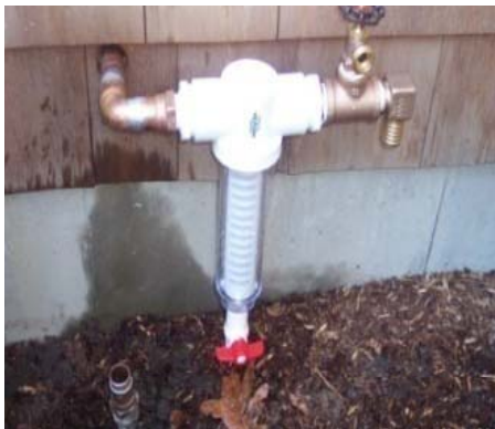
Clear View sediment filter with "Manual" flush valve for irrigation well (Wayland, MA)
