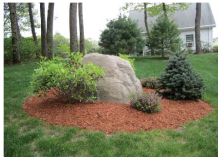
Well head covered with Artificial Rock and finished with landscaping Hingham, MA
