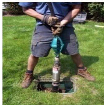
Pump Removal and Installations
