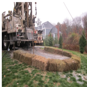
Debris Removal and Containment
