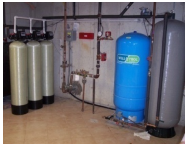
Large "Aeration System" for removal of iron in basement of residence (North Reading, MA)
