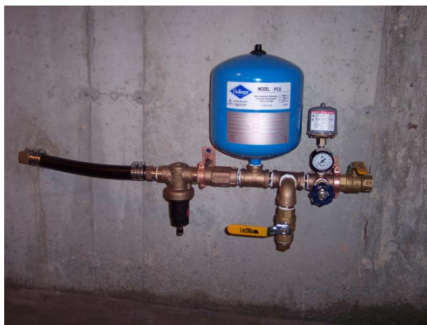
Mechanical Valve Constant Pressure System (CPS) in basement with port for possible future whole house use (North Reading, MA)
