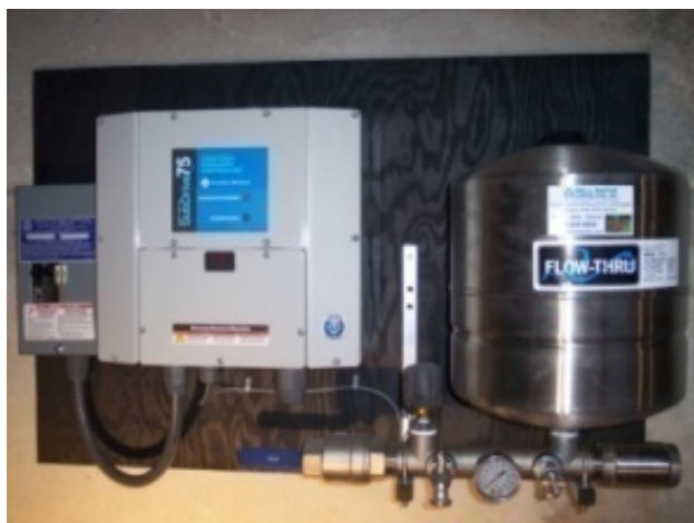
Whole House Variable Drive Constant Pressure System with stainless steel tank components and NEMA 4 controller mounted on board (Tewksbury, MA)
