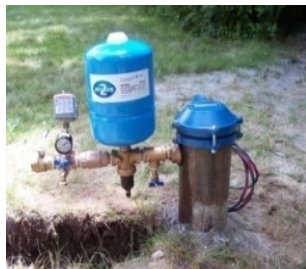
Artesian Well Submersible Pump System & Mechanical Constant Pressure System
