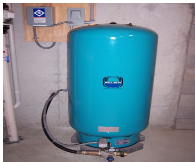
Traditional Whole House System with large storage tank in basement (Hingham, MA)
