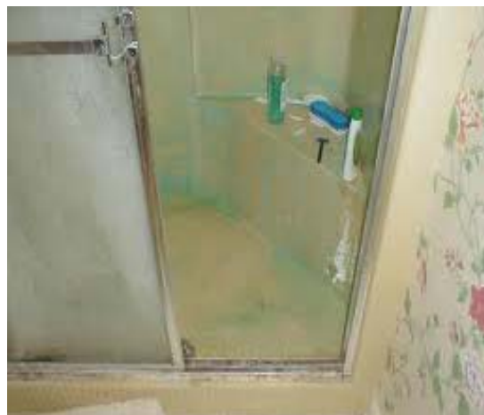
Visible Effects of Pipe Corrosion
