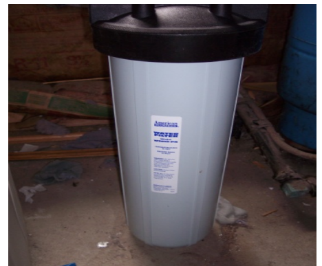
Cartridge Filter to remove sediment from well in whole house water system (Stoughton, MA)
