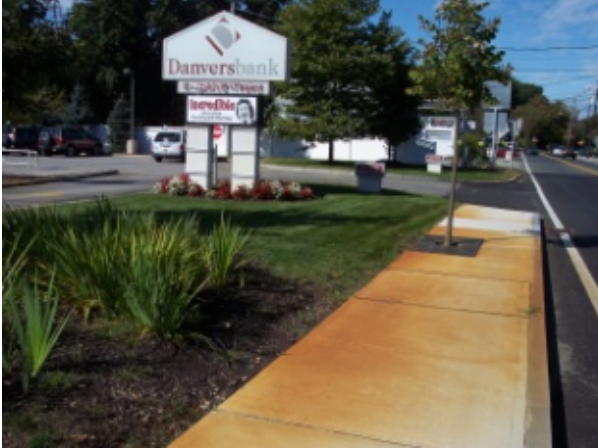
Heavy iron stains on sidewalk at commercial property before removal (Wilmington, MA)
