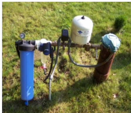
1 micron bag filter for removal of fine sand and silt from irrigation well (Hopkinton, MA)
