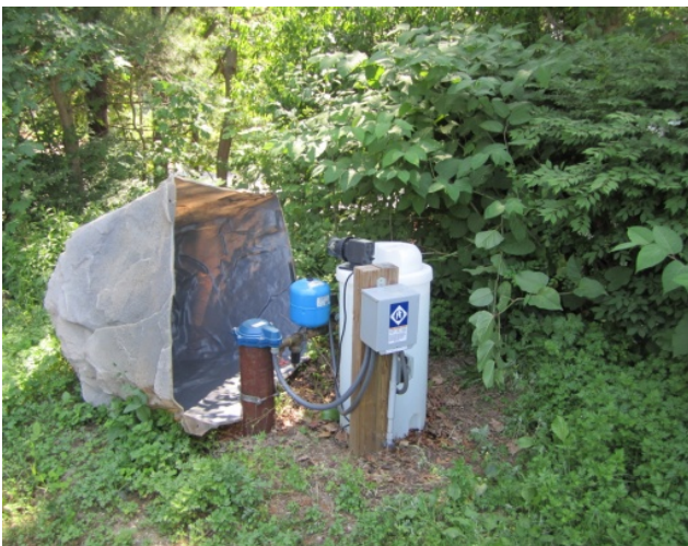
Stain prevention system with 30 gal tank under landscape rock at commercial condominium (Hingham, MA)
