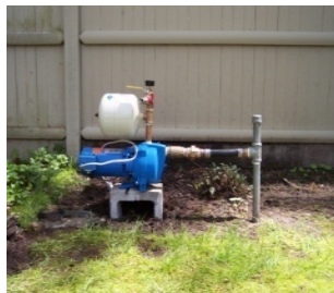
Shallow Well Jet Pump System & Tank System
