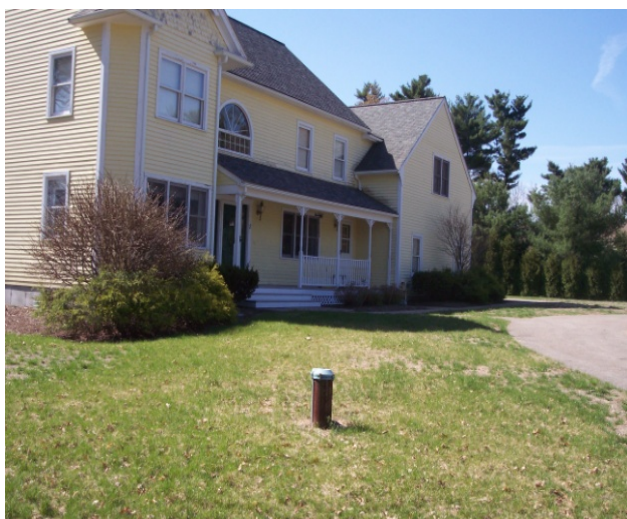
Whole House Well casing and cap ("well head") 18" above grade (Sudbury, MA)
