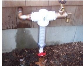
"Clear View" sediment filter with "Manual" flush valve (Wayland, MA)
