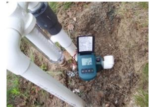
"Clear View" sediment filter including "Automatic" flush valve" (Canton, MA)
