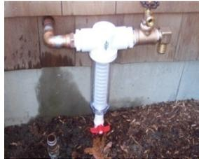
"Clear View" sediment filter with "Manual" flush valve (Wayland, MA)
