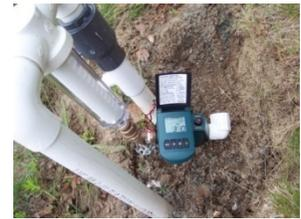
"Clear View" sediment filter including "Automatic" flush valve" (Canton, MA)
