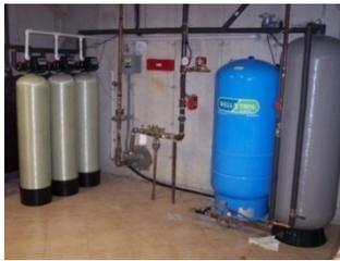
Large "Aeration System" for removal of iron (North Reading, MA)
