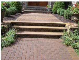
Front walkway showing iron stains from well water "BEFORE" stain removal process
