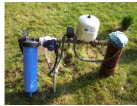
1 micron bag filter mounted after CPS for removal of fine sand and silt from well water (Hopkinton, MA)
