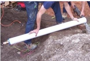
"Pump Screen" installed over submersible pump to limit intake of sediment (Wilmington, MA)
