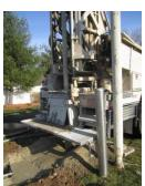
After the drilling, the pump gets installed inside the well casing and above the screen, and any additional components such as a tank system or sediment filter are also installed. An 18" deep trench is also needed to run electricity.
