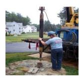
After the drilling, the pumping system is installed inside the well, and any additional components such as a tank system or sediment filter are also installed.
