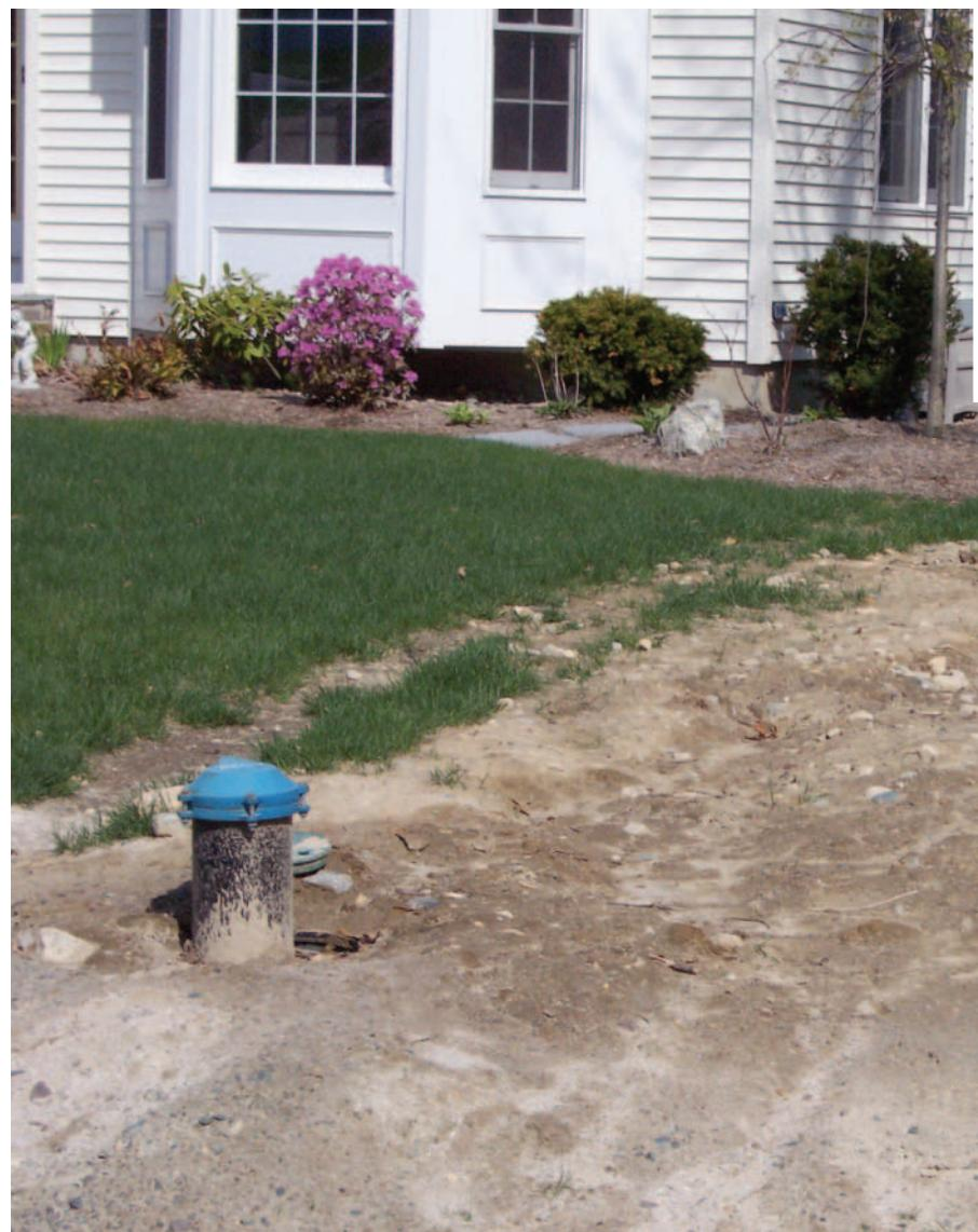
Completed well on the side of a home owner's driveway. Above right: Trench dug for electricity to power the irrigation well's pump.
