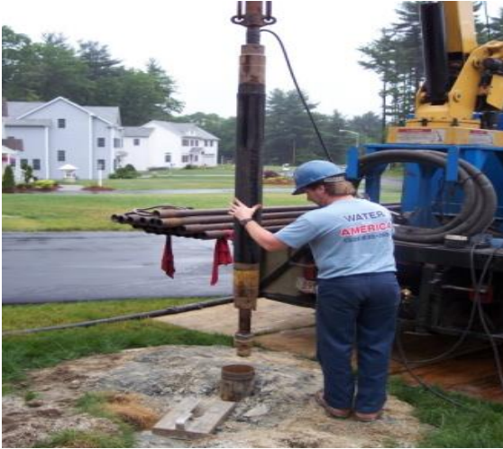
During hydrofracturing, a single inflatable packer is lowered into an Artesian well (Wilmington, MA)
