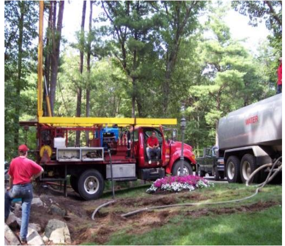
During zonefracturing two inflatable packers are used (Dover, MA)
