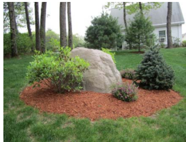
Well head covered with “Artificial Rock” and finished with landscaping.
