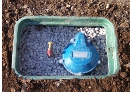
Well –head “Cut Below Grade” and installed in jumbo irrigation box with cover. (Wilmington, MA)
