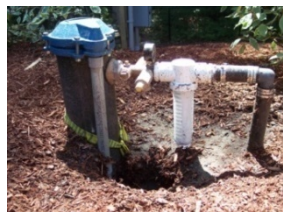
Tank-less Constant Pressure System for "irrigation only" (with no spigots) (Sharon, MA)
