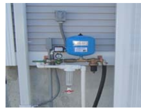
Constant Pressure System on side of house with electrical components and sediment filter. (Milton, MA)
