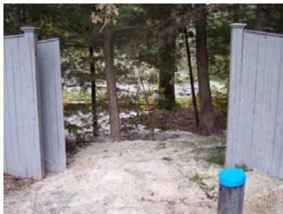
Removal of fence for access with equipment and/or allow for removal of drilling debris
