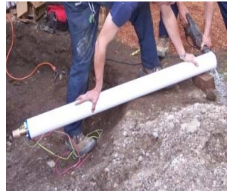
Pump Screen installed over submersible pump to limit intake of sediment from irrigation well (Wilmington, MA)
