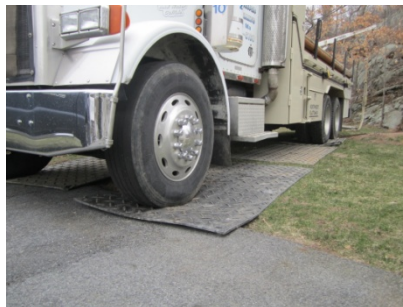
Delivery, use and removal of mud tracks for use on sensitive areas
