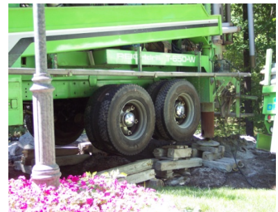
Provide blocking to support weight of heavy drilling equipment
