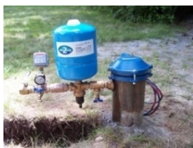
Constant Pressure System mounted to well, for hoses to garden, sprinklers and pool. (Franklin, MA)
