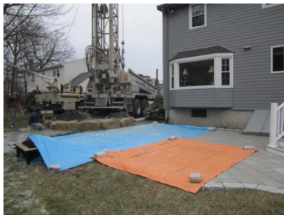
Use of tarps to prevent mud splatter on new blue stone patio
