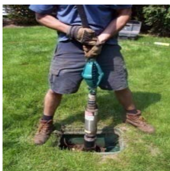
Pump Removal and Installations
