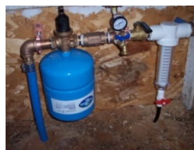
Constant Pressure System including filter and electrical components mounted in shed. (Wilmington, MA)
