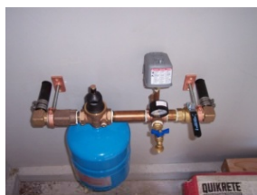
Constant Pressure System for sprinkler system mounted inside garage. (Wayland, MA)
