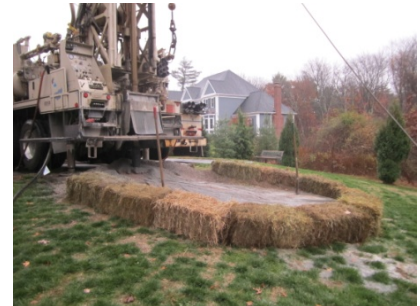
Delivery and use of hay bales to help divert or contain drilling mud
