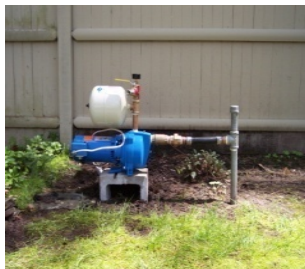
Shallow Well Jet Pump System & Tank System
