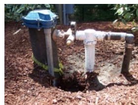
Tank-less Constant Pressure System for “irrigation only” (with no spigots) (Sharon, MA)
