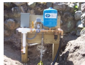
Constant Pressure System and controls mounted outside on pressure treated lumber. (Dedham, MA)
