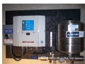
Variable Drive Constant Pressure System with stainless steel tank components and NEMA 4 controller. Mounted on board. (Tewksbury, MA)
