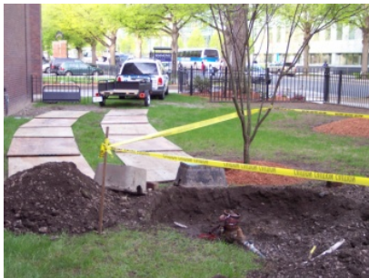
Delivery, use and removal of plywood for use on sensitive areas
