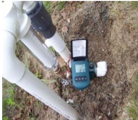
Clear View sediment filter including "Automatic" flush valve for irrigation well (Canton, MA)
