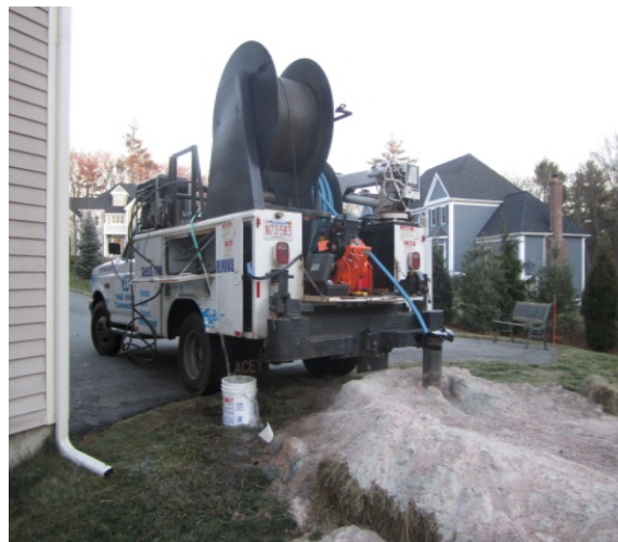
A pump test is performed afterwards to determine the new flow rate (North Reading, MA)
