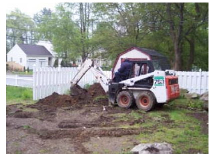
Use of equipment to level off ground to allow access and safe set-up of drilling rig
