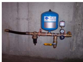
Constant Pressure System mounted in basement of home with additional port for future expansion. (North Reading, MA)
